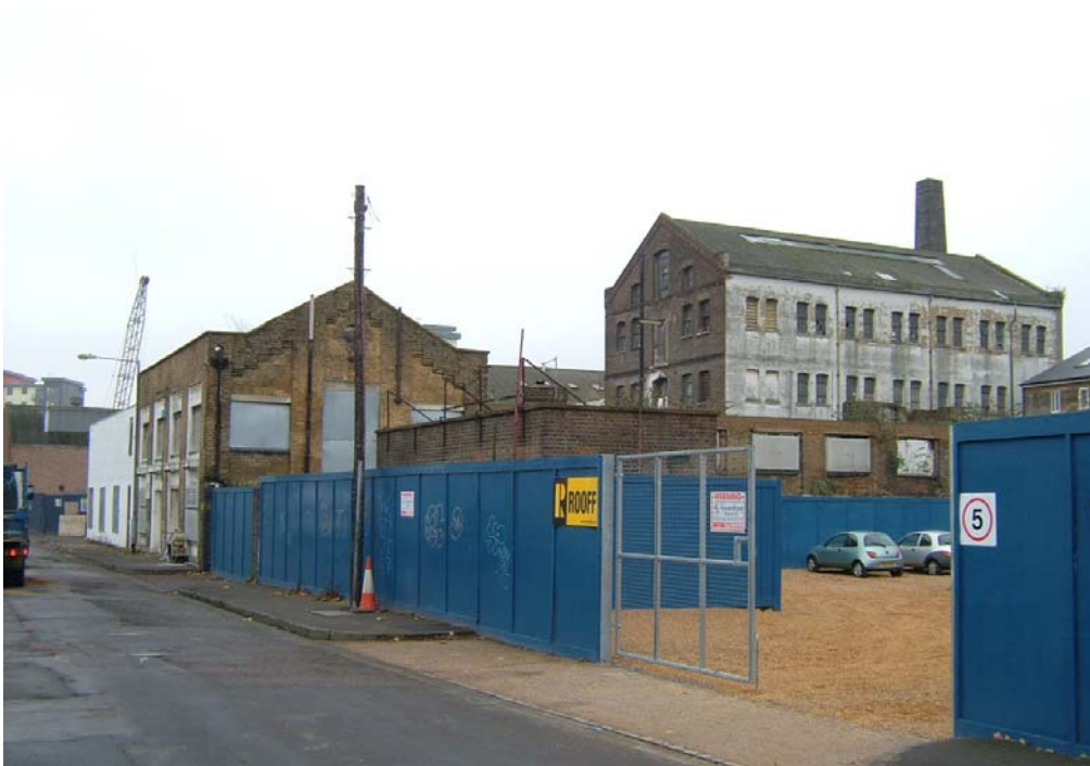
Figure 28 the two storey Malthouse Extension before it was demolished (Granary the taller building behind) (source: the writer)
