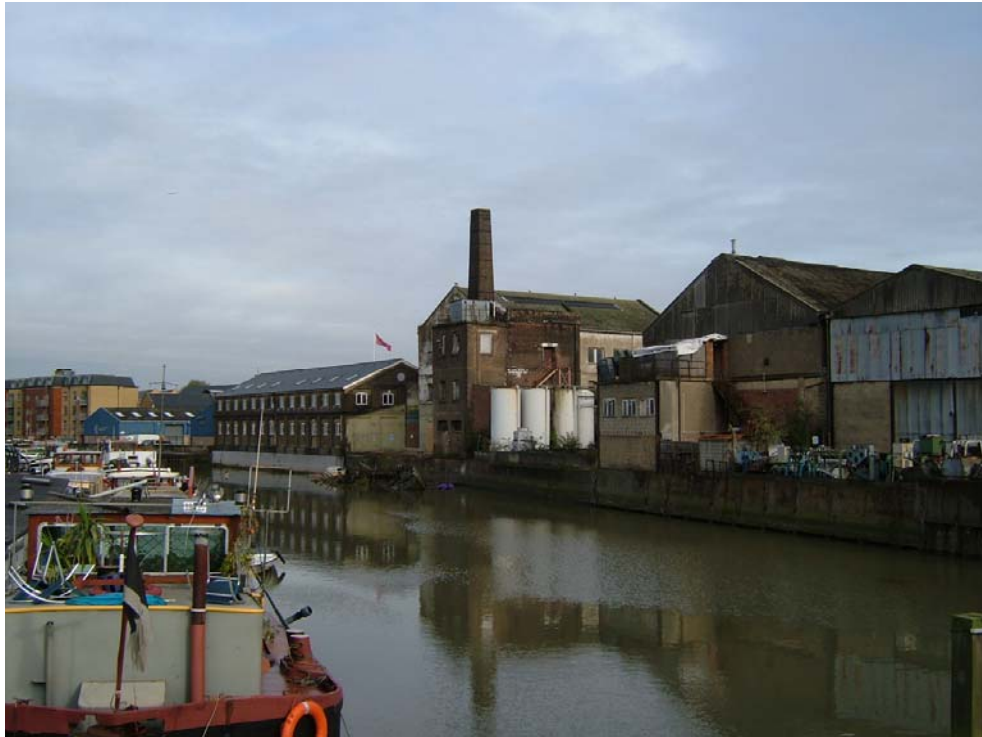
Figure 15 access to the barrage has recently been made available which provides a good view of the Malthouse and Granary (source: the writer)
