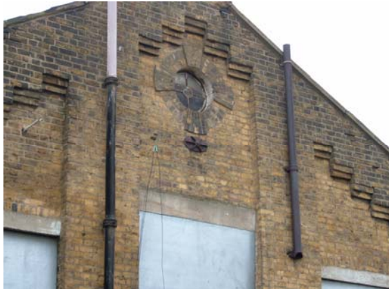
Figure 35 the gable ends now demolished which were on the Malthouse Extension (source: the writer)
