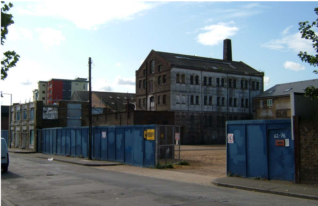
Figure 17 view of the conservation area today from Abbey Road showing the Malthouse and Granary building as the main remaining features (source: the writer)
