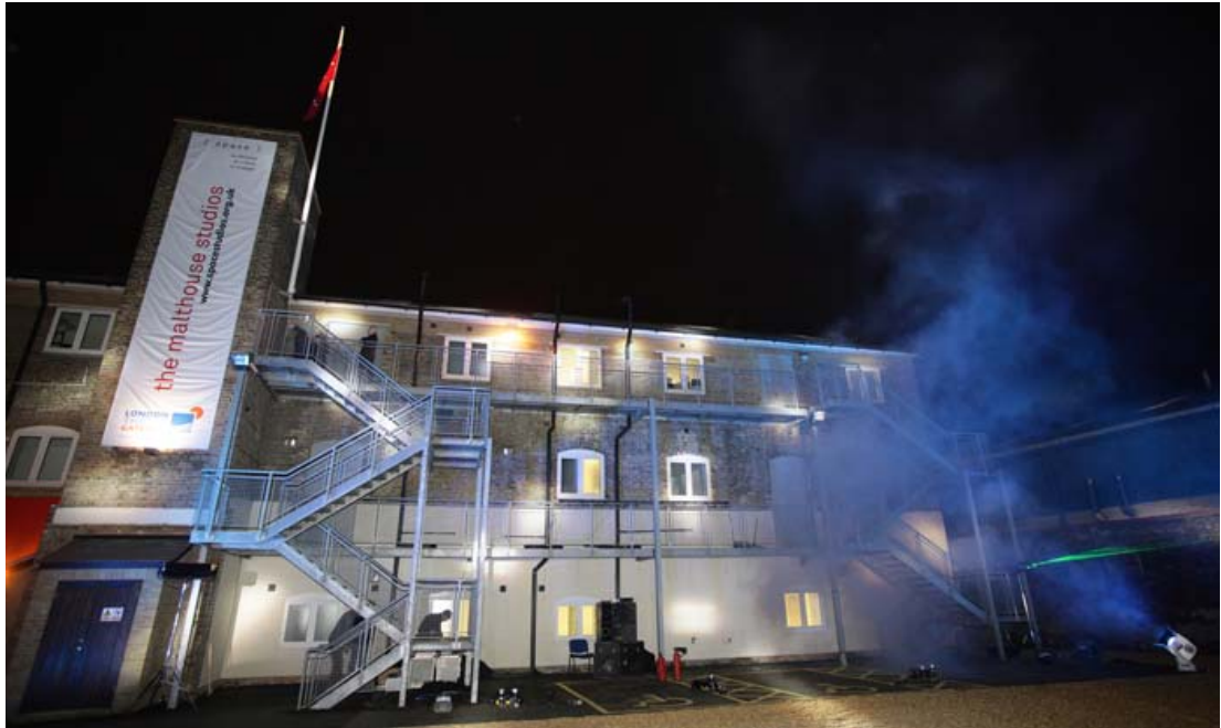
Figure 5 the Malthouse refurbished as part of the Creative Industries Quarter (source: LTGDC)
