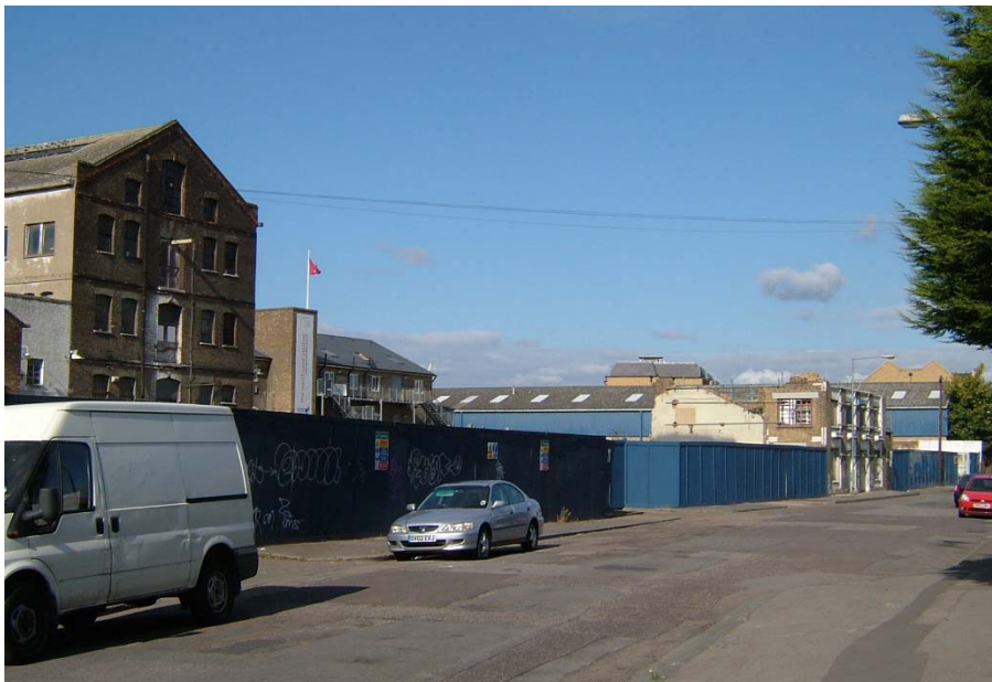
Figure 30 showing the façade of the barley loft on Abbey Road (source: the writer)
