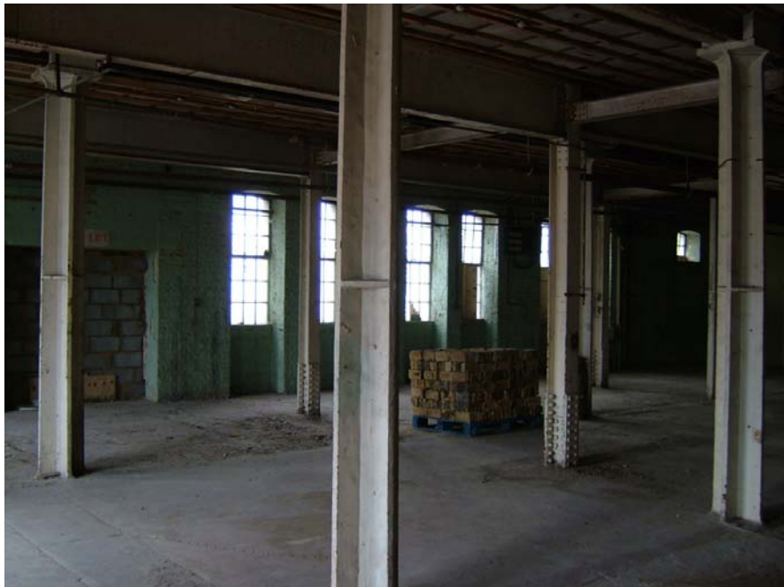
Figure 24 the interior of the Granary remains intact (source: the writer)
